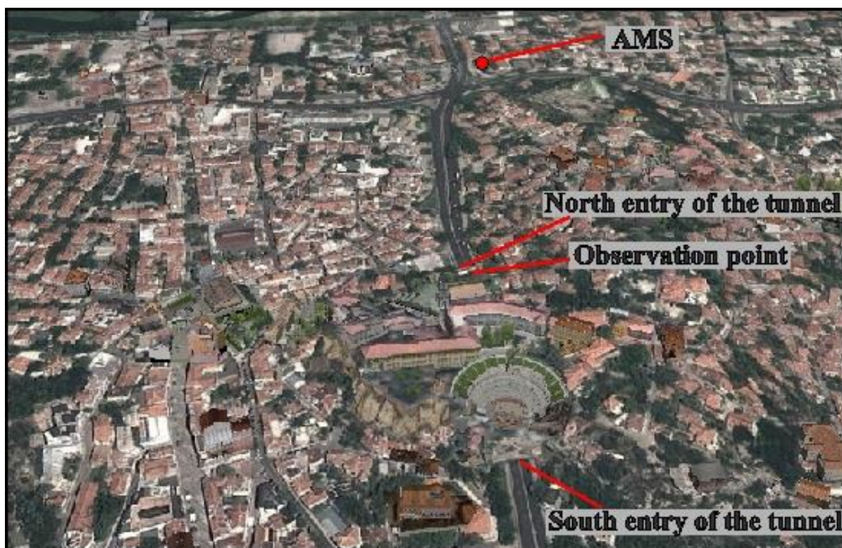
Fig. 1. Satellite picture of the transport tunnel in the city of Plovdiv, Bulgaria (source Google Earth, 2014), location of the observation point and of the automatic measuring station (AMS)
