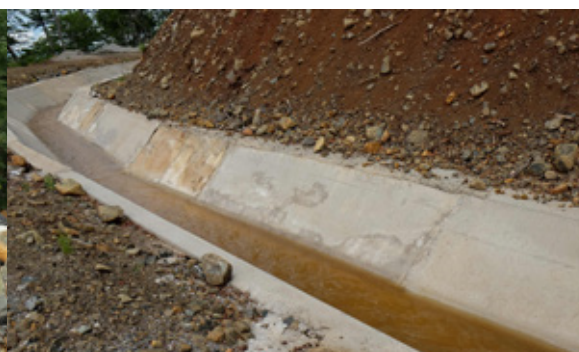
Figure 15: Feeder channel bringing sediment into Liqeni i Zi
