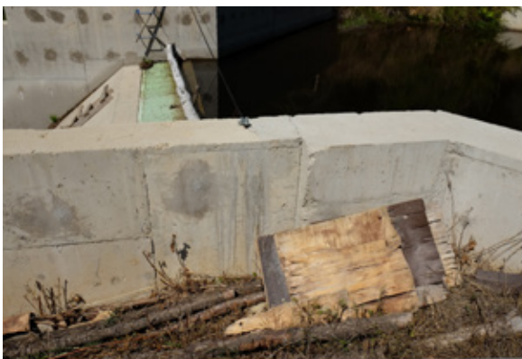
Figure 22: An appliance potentially used for blocking the fish pass on Stanisar intake
