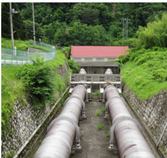
Figure 4: Pipes entering the powerhouse of a derivation plant. Author: Qurren Figure 5: Ilovac run-of-the-river plant, source: TSREDCO Ltd.
