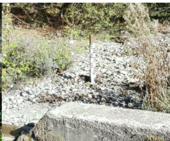
Figure 27: The weir above the powerhouse November 2017
