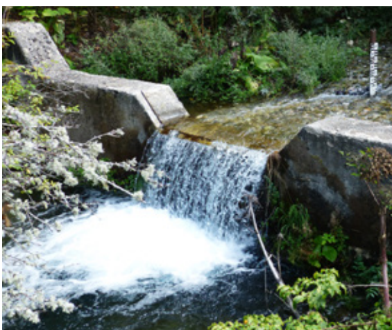
Figure 26: The weir above the powerhouse September 2017
