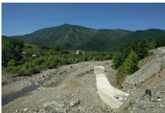
Figure 10: Tunnel taking tailwater to Rapuni 3 & 4
